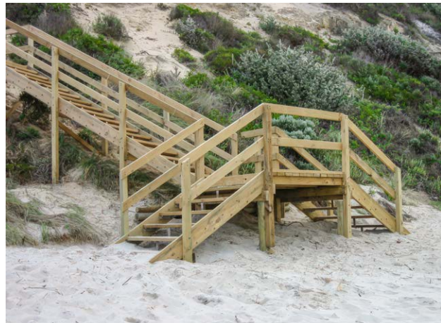
Salmon Holes, Torndirrup National Park. Photo: DBCA.
